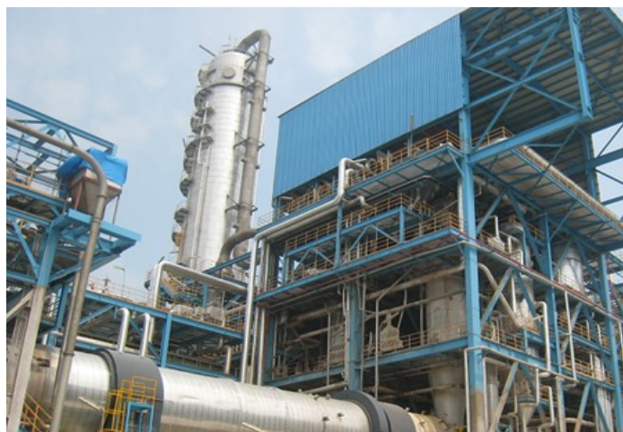
Photo 1: Typical chemical manufacturing plant.
